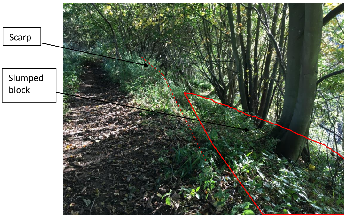
Plate 3.5 Stop 11 (approx. Ch. 12800m) View from the footpath on the north side of the River Coquet looking south east.
