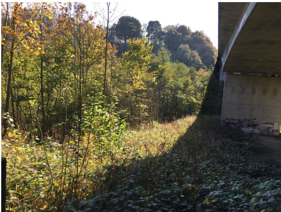
Plate 3.8 Stop 11 (approx. Ch. 12800m) View south of the River Coquet Bridge piers from the footpath on the North Slope.
